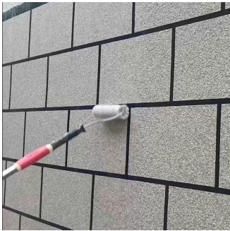
04. Sand with 320-grit sandpaper, and then roll coat (spray) topcoat 1-2 times, each time interval 4-6h (23±2°C)
