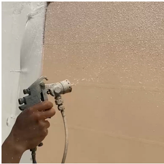
03. Spray Granite Paint 1-2 times evenly with a special spray gun (caliber 3.0-4.0), each time interval 8h (23±2°C)
