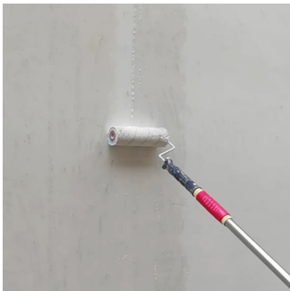
01. Roller primer(or black primer) 1~2 times, each time interval 6h (23±2°C)
