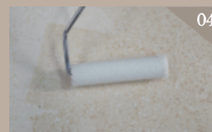
Cover layer (recommended to use ultimate matte cover) uniform Roll coating twice (add 10-15% water)
