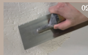
Batch once, control to ensure uniform particle thickness After semi drying, let it shine until the surface is smooth
