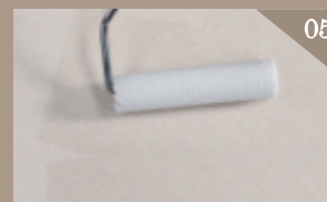
Cover layer (recommended to use ultimate matte cover) uniform Roll coating twice (add 10-15% water)
