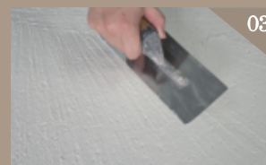
After drying thoroughly, use 180 grit sandpaper or a shovel to remove the protrusions Scratch the second time
