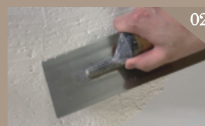
Use a stainless steel scraper to scrape the first layer of the main material (Thickness of about 1mm)
