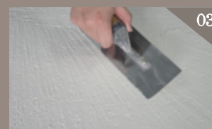
03 After drying thoroughly, use 180 grit sandpaper or a shovel to remove the protrusions Batch 2
