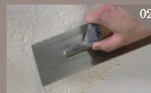
02 Scrape a layer of main material with a stainless steel scraper (Thickness of about 1mm)
