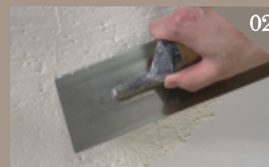
Adjust the water addition ratio according to the temperature during construction Batch 2 times
