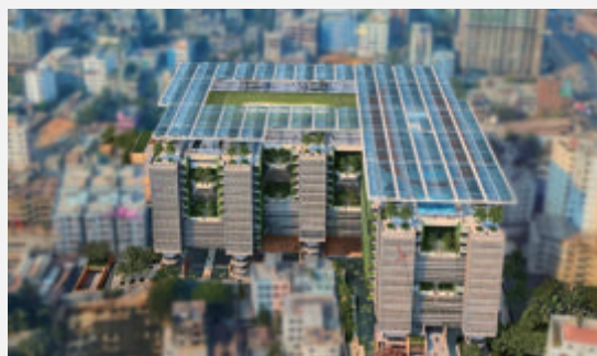
PROJECT : BRAC University New Campus - Bangladesh
